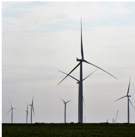
Rock Falls Wind | EDF Renewable Energy
